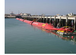
(iii) Pelamis Wave Energy Converters in the harbor of Peniche, Portugal
